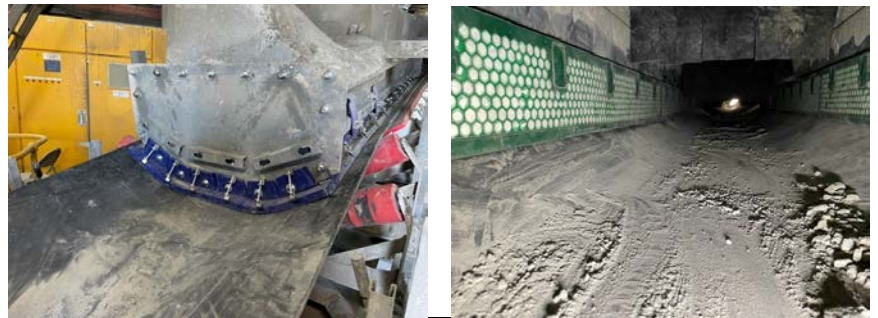
Photos: After Installation of TailScrape (L) and K-Containment® Seal (R)
